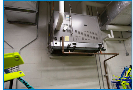
Gas-to-Steam (GTS ® ) humidifier presiding over a room full of freshly painted Project One bike frames. Steam from this unit is ducted to the finishing room.
