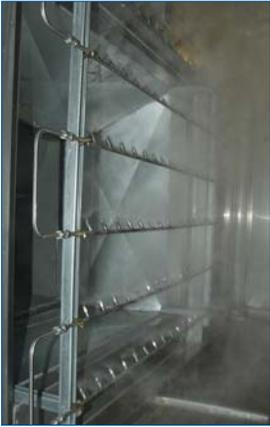
**Minimal maintenance.** Adiabatic humidifiers using reverse-osmosis-treated water (RO) or deionized water (DI) require the least maintenance. Adiabatic systems that use tap water require cleaning or component replacement to remove deposited minerals. Systems with moving parts (humidifiers with rotating disks and atomizers with movable nozzle pins) require periodic parts replacement.
